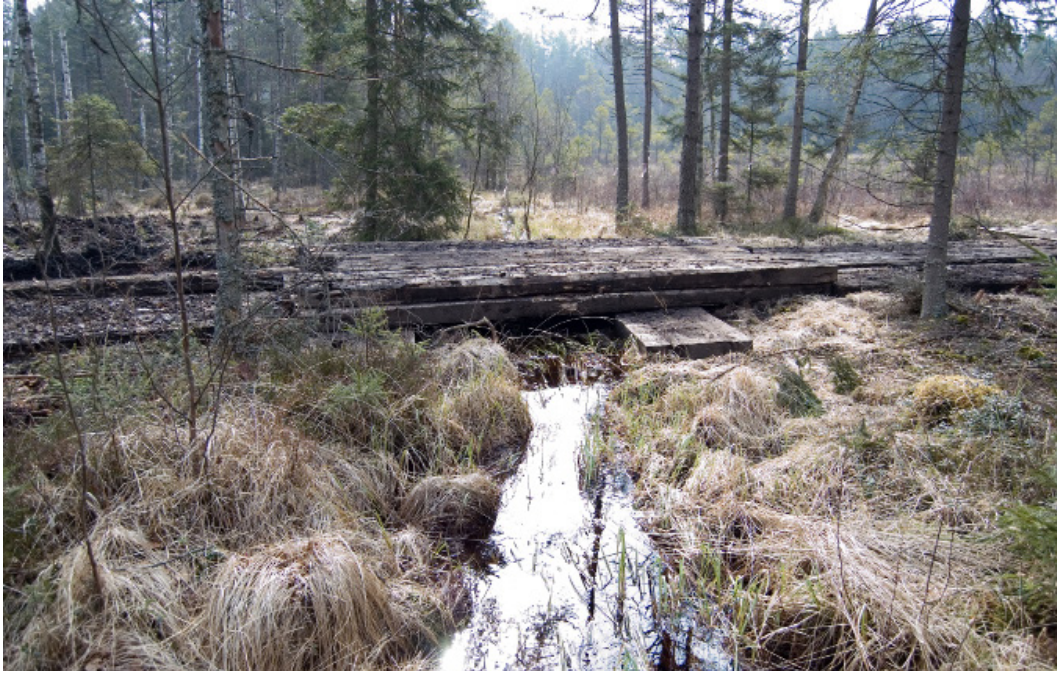
Fig. 9. An example of a temporary bridge. Photo by Eva Ring.
