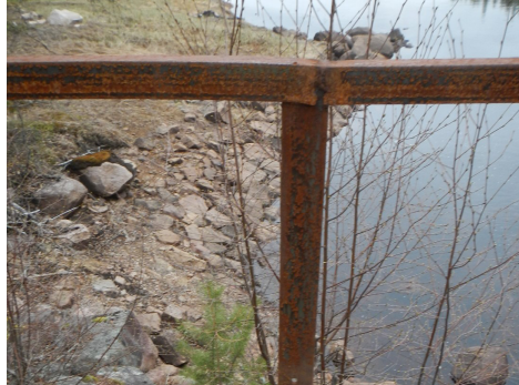
Räcke - Korrosion/Deformation.
