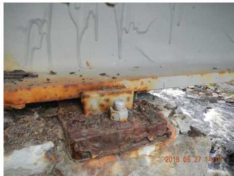
Lager - Korrosion.
